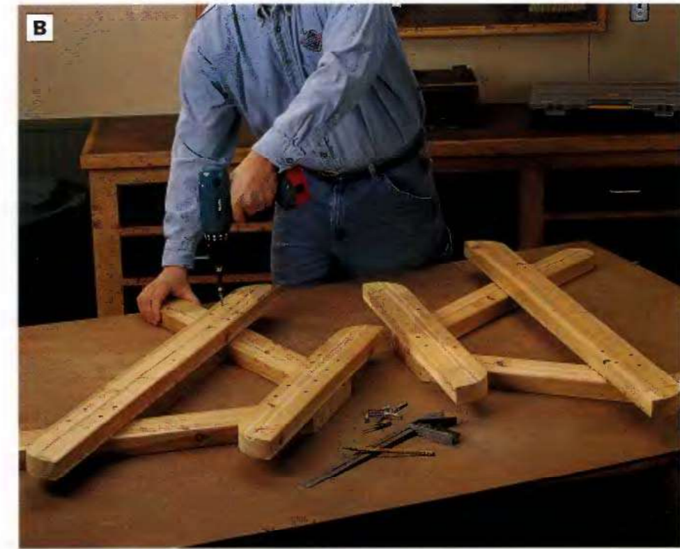
PHOTO B: Set pairs of legs on your worksurface so they splay outward with their angled ends aligned. Attach the top stringers flush to the tops of the legs, and install the seat stringers so they overhang the legs by 8 in. on each end. Fasten the parts with countersunk 2 1/2-in. deck screws to form two leg assemblies.
